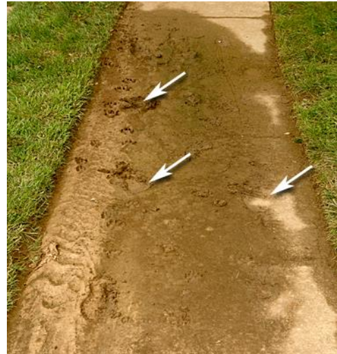
Figure 1. On this muddy sidewalk, skid marks (indicated with arrows) show where people slid.
