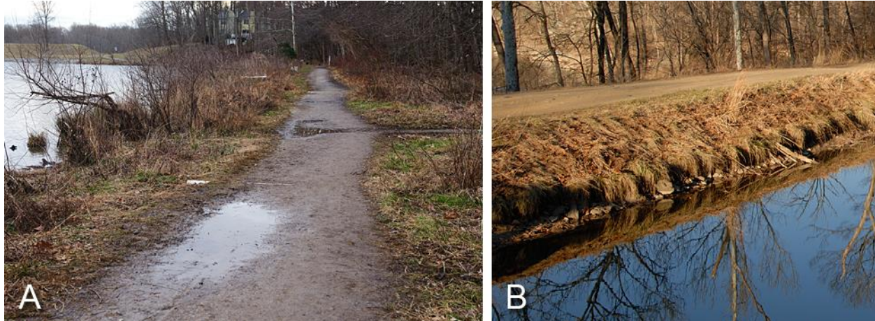
Figure 4. People love walking next to lakes and rivers. However, trails adjacent to waterways with elevations close to the normal water level end up muddy (A). The water table under the path is close to the surface. Any precipitation does not absorb into saturated soil and is unable to readily drain off the flat terrain. Four-inch PVC tubes meant to facilitate drainage are inadequate and wind up clogged. When winter arrives and the water freezes, ice expands and heaves the trail. This western section of Royal Lake's loop receives some of the most complaints about mud because it is placed in an inappropriate area, requires much up-keep, and is an unsustainable trail section. Putting the trail along the nearby slope would be a better location. Examples of sustainable, natural-surface trails next to water include the C&O Canal towpath at Great Falls National Park (B) and paths along bedrock, such as Great Falls' Billy Goat Trail (not shown).
