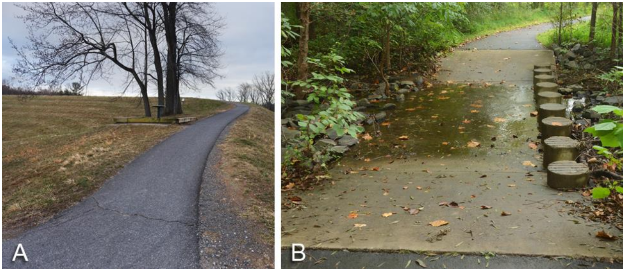
Figure 3. Paved trails have their place, such as to ADA-accessible venues and sport fields. Asphalt trails are necessary across artificial structures such as dams and spillways (A). Concrete is used in small, specialized trail sections like stream crossings (B) where water flows over the part for maintenance vehicles and dry steppingstones enable pedestrians to transverse. Concrete crossings are expensive and used in select locations.
