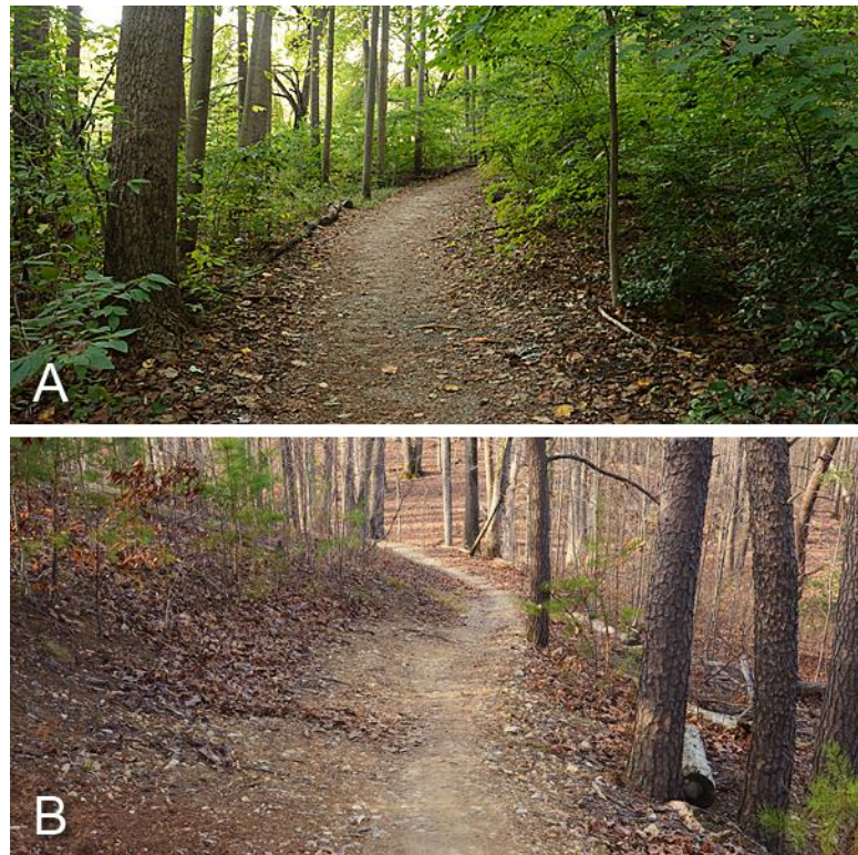
Figure 1. Most Fairfax County trails were created before sustainability became a consideration. Some of these trails, such as this clay and stone footpath along a well-drained forested hillside (A), happen to be sustainable. Such natural surface pathways are easier on the knees than pavement. Many new, natural surface hiking and mountain bike trails (B) are created with sustainable designs.
