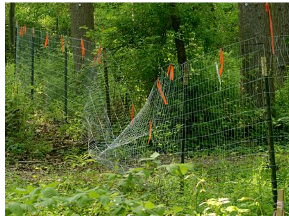
Figure 3. Welded wire fences encircling the LOD are to protect folks from construction activities. This example of vandalism is doubly selfish because it occurred on an unauthorized path away from the main trail.
