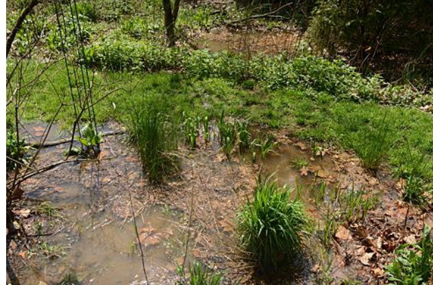
Figure 3. The primary rain garden (front) and a secondary one (back tier), are full after a heavy rain in early spring. Since all of this water will be absorbed within 24 hours after the last raindrop falls, the properly designed rain garden will never breed mosquitoes.
