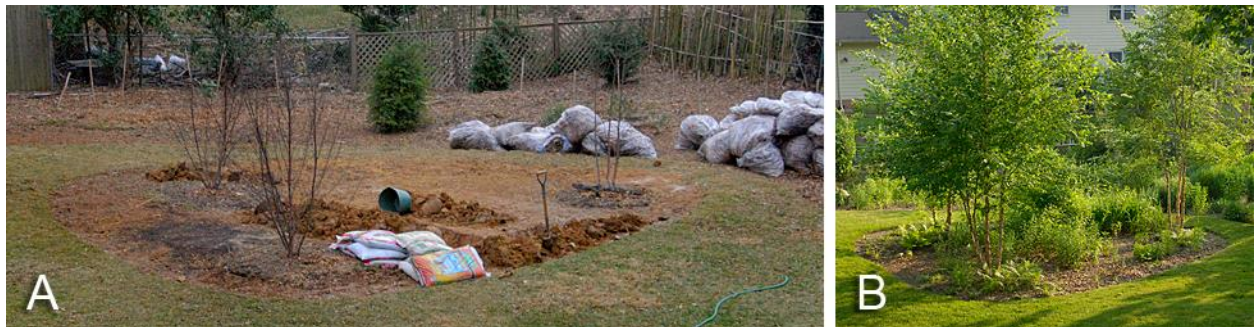
Figure 2. This rain garden's construction is near completion (A). Three river birch saplings are planted at least 15 feet apart and the last of the soil amendments are added. Photographed in March, the leaf bags resting on the berm were donated by neighbors back in autumn. Two years after installation (B), the rain garden's plants grow into the plot.
