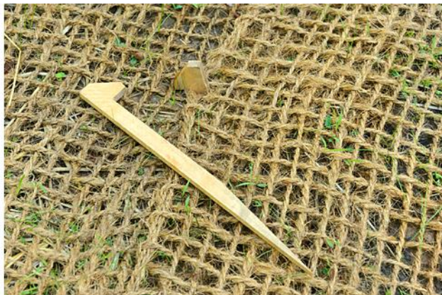
Figure 7. To help the grass grow, scattered straw on bare ground is held by a biodegradable coir net. Wooden stakes secure the net, which protrude and therefore are used away from traipsing hikers.
