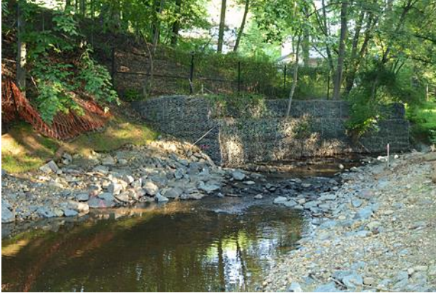
Figure 8. The restoration's upstream terminus (left) used modern approaches to replicate a natural creek. It is a more conducive environment for aquatic life than the gabion walls (center) to control bank erosion, which were installed decades earlier. This wall and the concrete-lined portions of creek bed with "speed bumps" (not seen here) are outdated waterway control methods.
