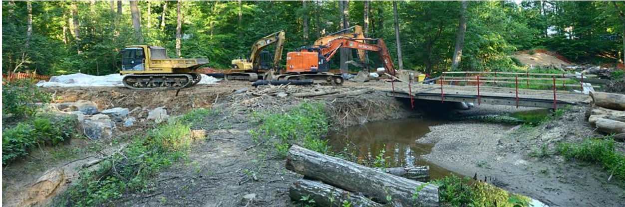
Figure 3. A temporary bridge enabled earthmovers to cross Rabbit Branch and perform work upstream. Boulders on the left await placement in repairing the water's course from a storm drain outfall. Logs from fallen trees (center) will integrate into the stream bank and provide favorable habitat for aquatic life.
