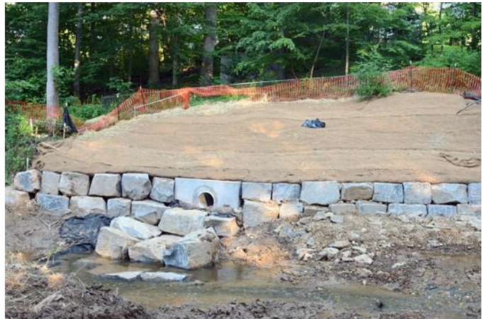
Figure 2. The “after” shot of the restored area shows a new outfall where stormwater hits stone boulders. A rock wall protects the hill from churning floodwaters. Until native restoration plants arrive, coir and straw promote grass growth that retains the soil. The county and other institutions are getting away from synthetic lawn netting since it inevitably becomes another source of plastic waste polluting the environment.
